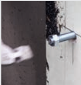
Drive heavy-duty dowels halfway into concrete wall
