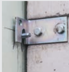
Hanging the light well to the dowels
