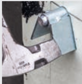
Hammering in the fastening element
