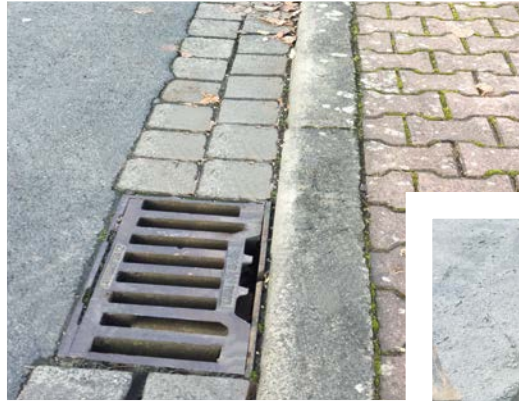
SITUATION BEFORE INSTALLATION
