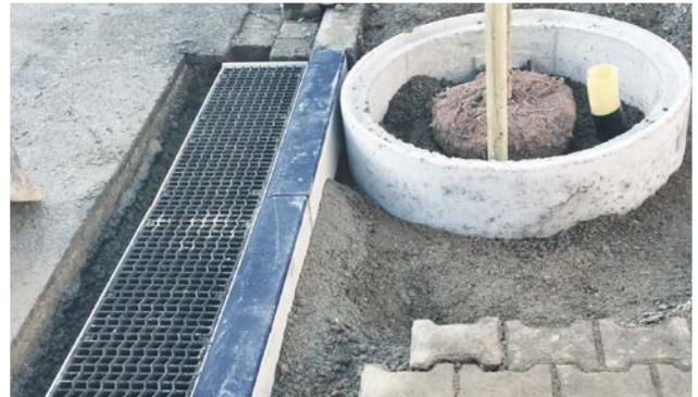
MEACLEAN PRO DURING THE INSTALLATION PHASE
