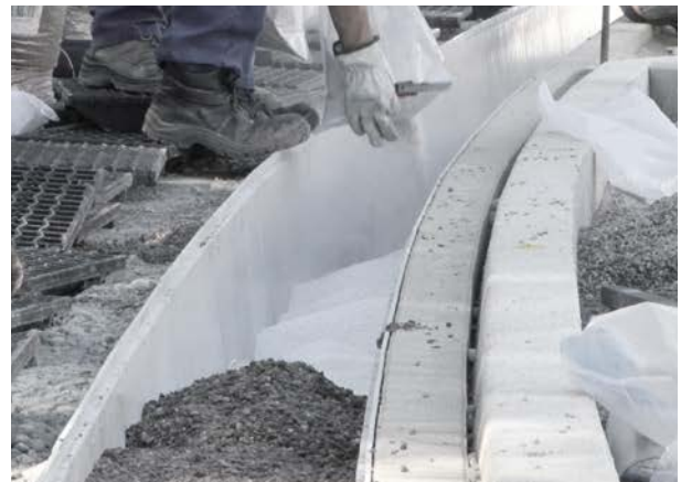
Step 2: Fill in and level-off the first substrate layer "Biocalith K".
