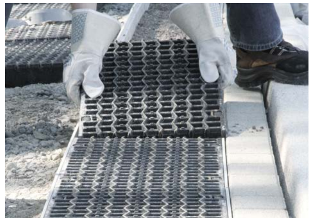
Step 4: Covering the channel strands with MEA gratings
